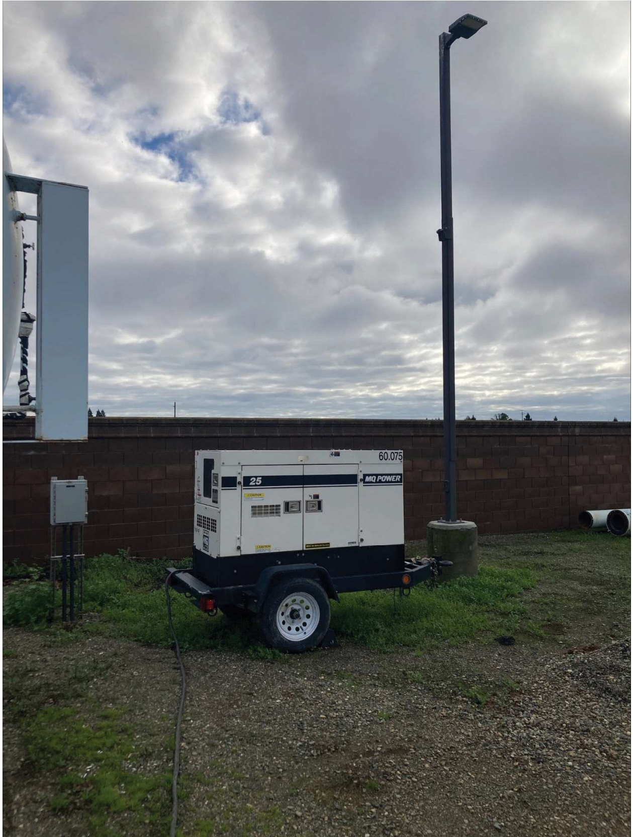
View of location of placement of New 80' Tower, facing East (ignore portable generator, will be removed)
