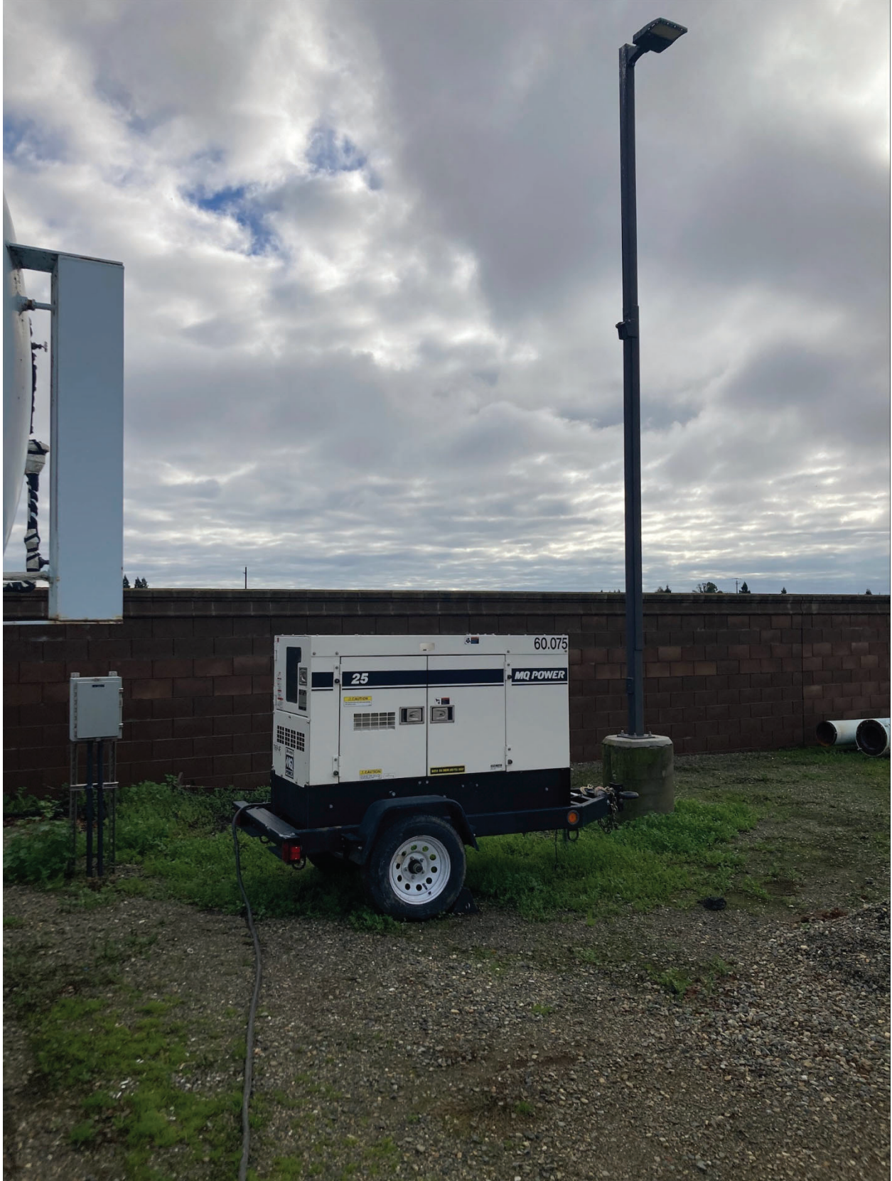
View of location of placement of New 80' Tower, facing East (ignore portable generator, will be removed)
