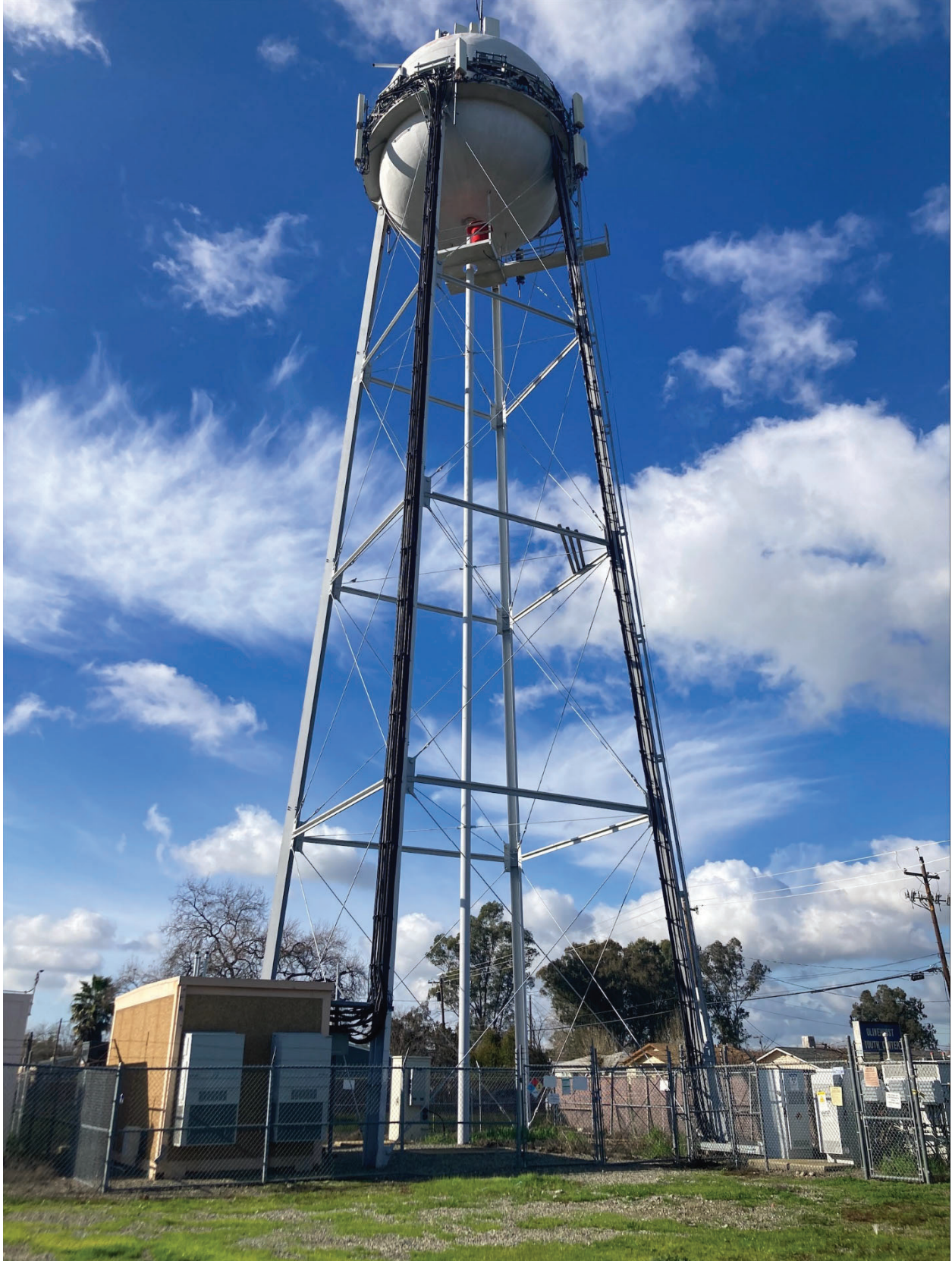
Aerial view of Existing Tower Location (Facing NorthWest)
